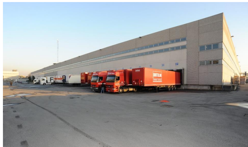
Outside of the warehouse in Cavenago
